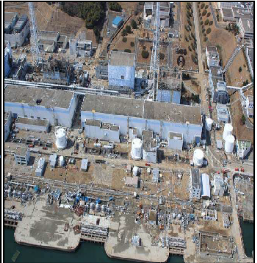
After the Earthquake and Tsunamis
